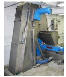
The cleaning system is made of a rake with a perforated collecting spoon capable of removing the captured particles conveying them toward the outlet. A wiper will completely remove the solids from the spoon. The cleaning system is operated by 2 roller chains driven by a single gear motor.
