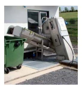
The following part is the transport zone, where the screenings free of organic matter are conveyed; at the end of the transport module the drain module completely eliminates the liquid residues coming from the washing zone, repeating the waste washing a second time.
